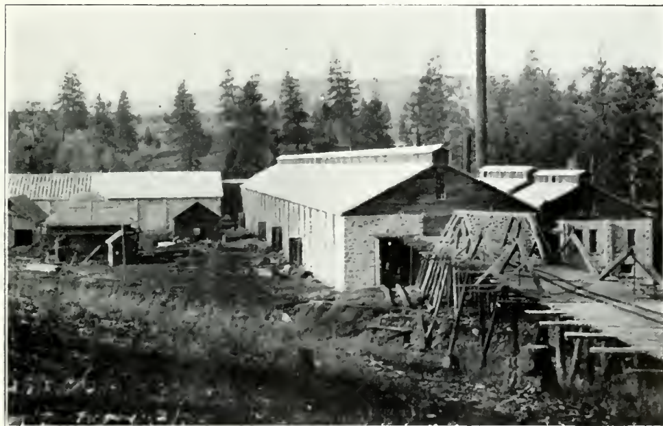
Cement-works under Construction at East Princeton.
